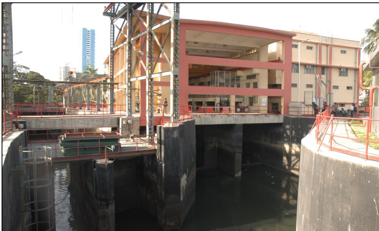
Haji Ali Stormwater Pumping Station
