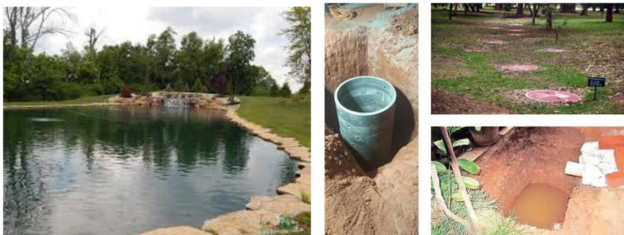
Fig 10.1 Recharge structures for RWH in Parks
