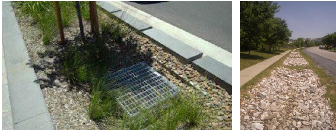
Fig 10.4: Infiltration Trenches along Roadside
