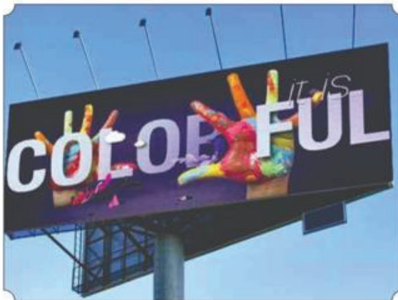
"V" Shape Hoarding
